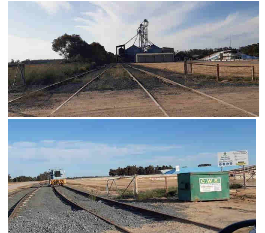
Figure 33: Photos of the GrainCorp Site & rail siding(s) (October 2023).
