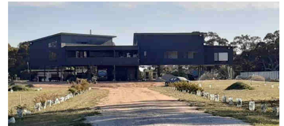
Figure 77: Example of a house outside the flood levee that has raised floor levels at additional expense.
