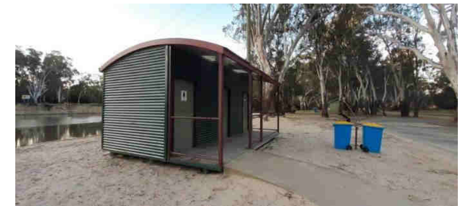
Toilet block/change rooms near main beach area.
