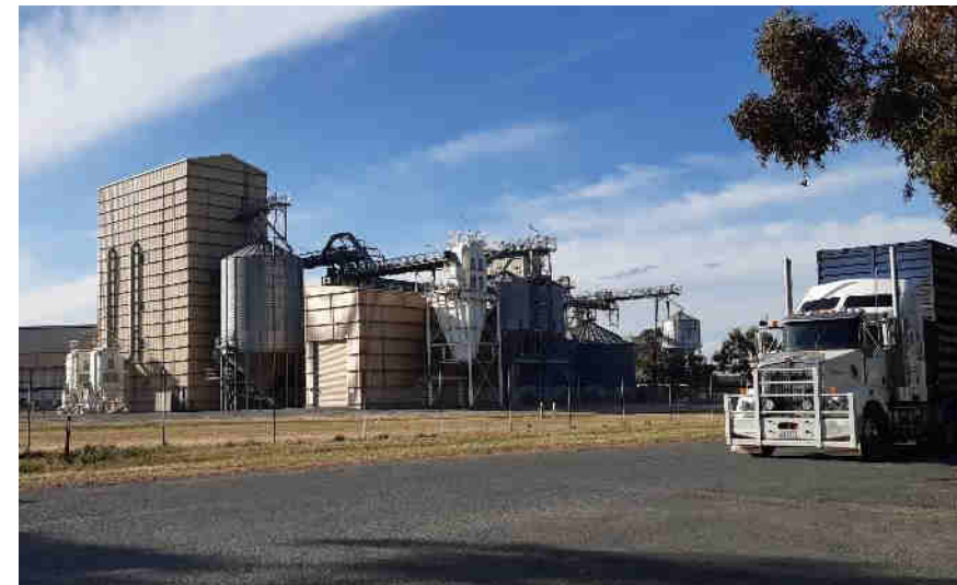
Figure 18: Photo of Sun Rice facility (October 2023).
