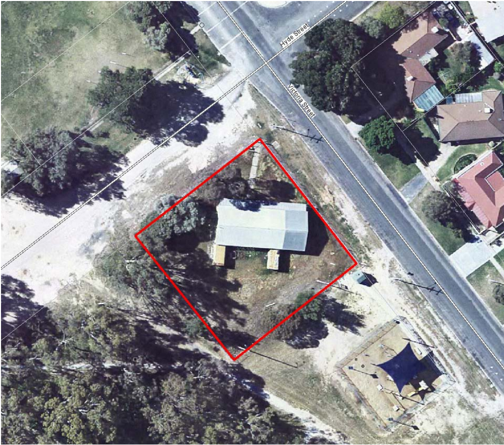
Figure 3 – Aerial Photograph of Former Scout Hall Reserve (Reserve No. 92579)
