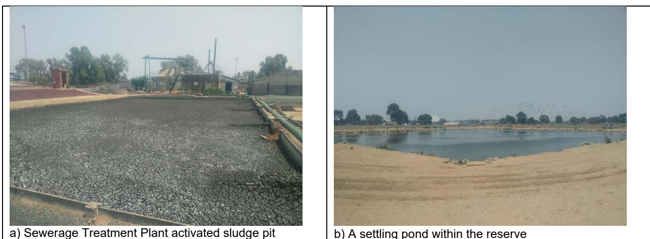
Figure 8 – Photographs of Sewerage Treatment Plant.
