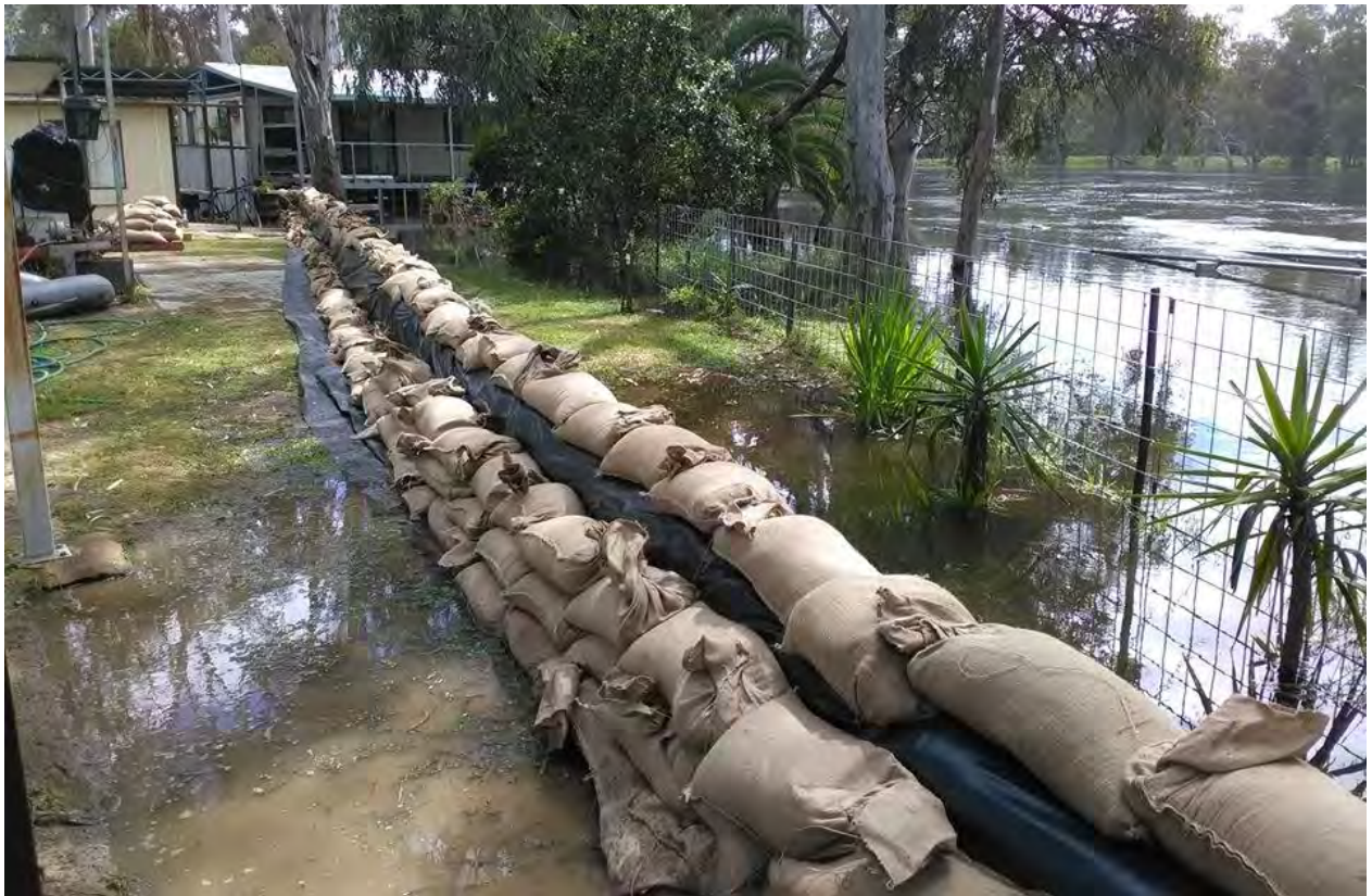
Photo 1 Sandbagging at McLeans Beach Caravan Park
