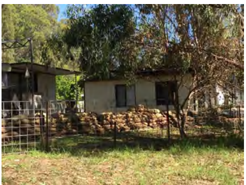
McLeans Beach Caravan Park Levee
