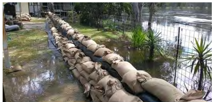
ABOVE: Sandbagging at McLean Beach Caravan Park.
