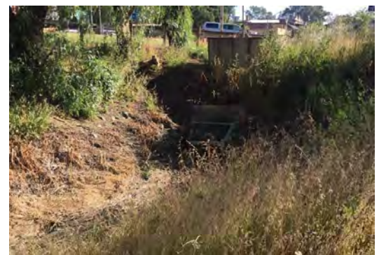
Pipe through South Deniliquin Levee
